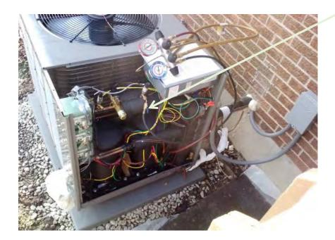
Field testing in OH-outdoor unit, at a residential home having a design cooling load of 3-ton (10.6 kW)
