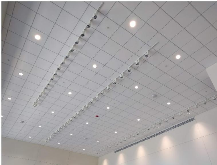
Figure 25. High LPD with Excessive Amount of Track Spotlights
