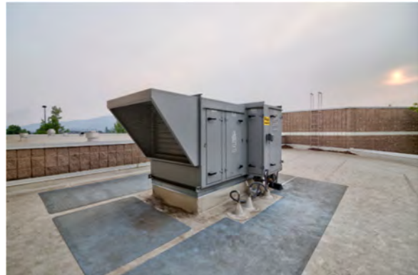
C-RTU INSTALLED
