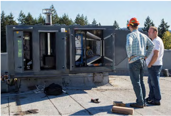
NEW UNIT INSTALLATION
