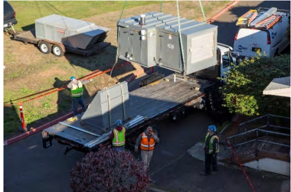
REPLACEMENT C-RTU CRANE PICK
