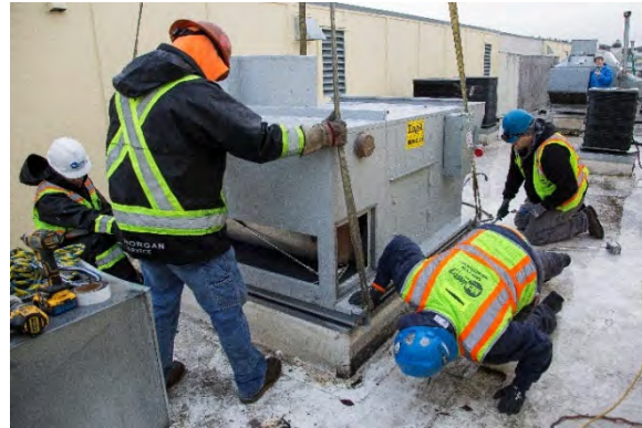
REPLACEMENT C-RTU PLACEMENT
