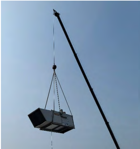
EXISTING UNIT BEING REMOVED
