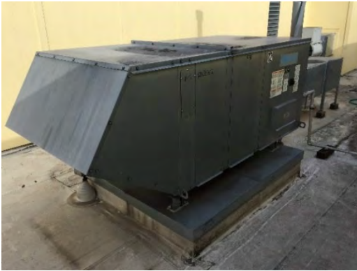
NEW C-RTU INSTALLED
