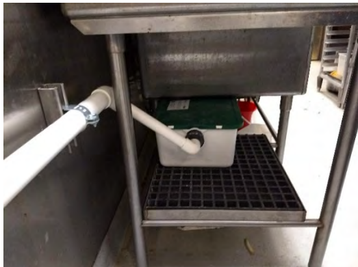
CONDENSATE NEUTRALIZER TANK
