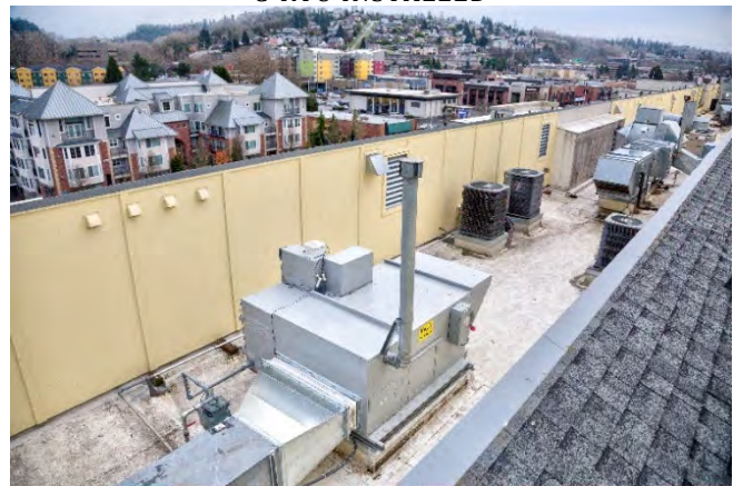
C-RTU INSTALLED
