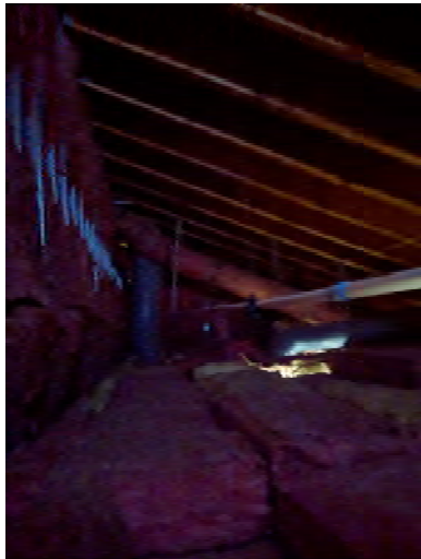
CONDENSATE DRAIN RUN IN ATTIC
