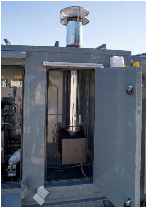
FIGURE 26 – FLUE BEFORE EXTENSION INSTALLED
