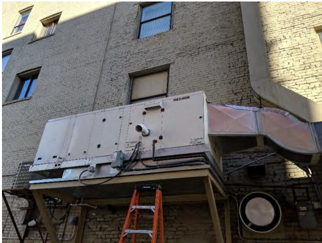
SITE D UNIT INSTALLED ON PLATFORM
