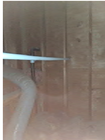
UNNEUTRALIZED CONDENSATE PENETRATION IN TOILET VENT PIPE
