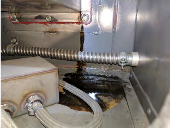
FIGURE 18 – SITE A FLUE BOX LEAK
