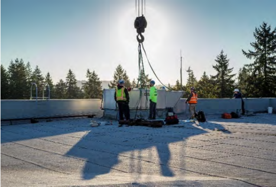
PREPARING EXISTING UNIT FOR REMOVAL
