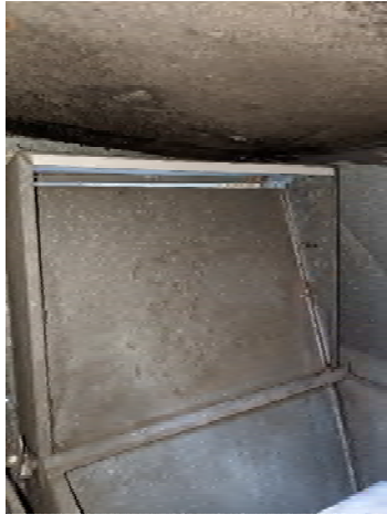
OUTSIDE AIR DAMPER CLOSED
