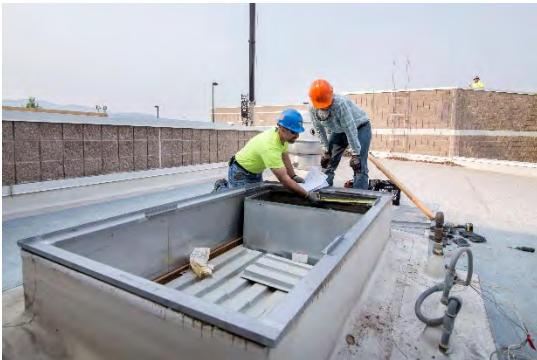
UTILIZING EXISTING ROOF CURB WITH CURB ADAPTER
