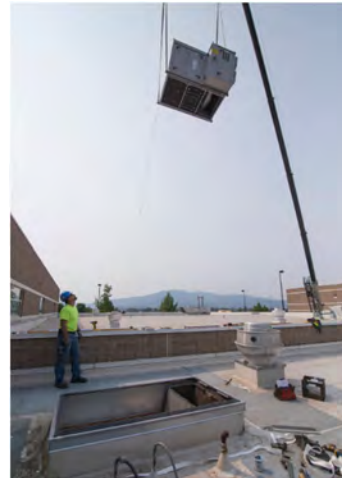
REPLACEMENT C-RTU CRANE PICK
