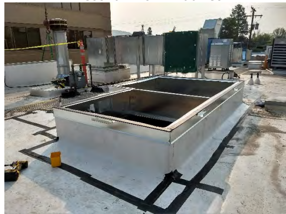
NEW CUSTOM-BUILT ROOF CURB
