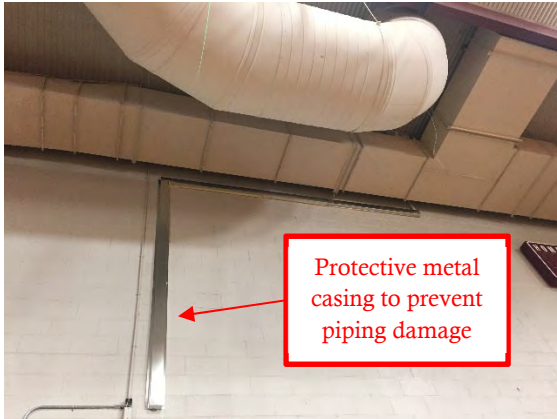
DRAIN PIPING WITH PROTECTIVE CASING
