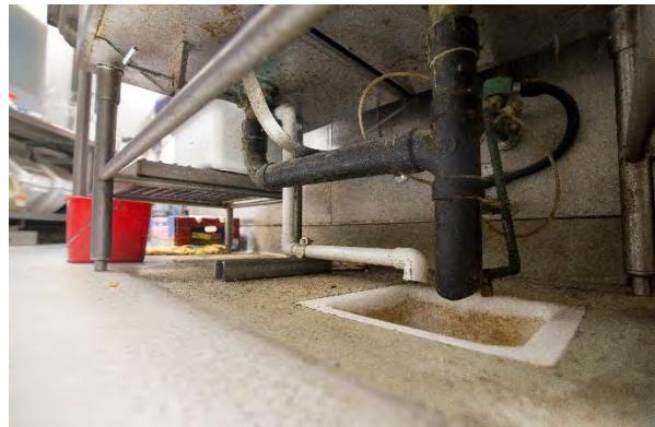
CONDENSATE DRAIN TERMINATION
