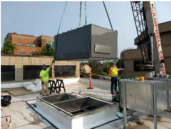
C-RTU CRANE PICK
