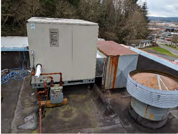
SITE B CONDENSING UNIT
