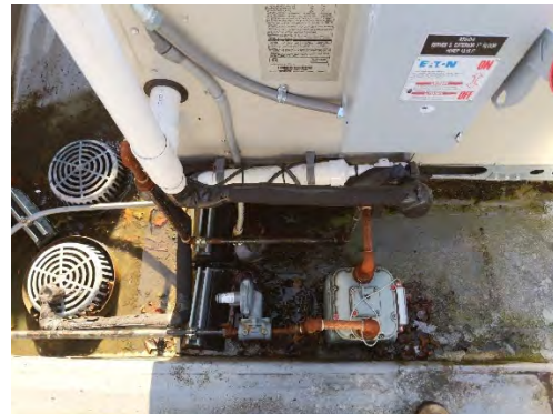
CONDENSATE NEUTRALIZER & HEAT TAPE
