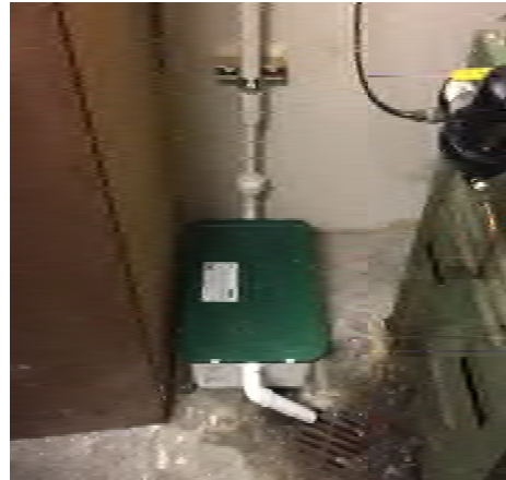
CONDENSATE NEUTRALIZER INSTALLED
