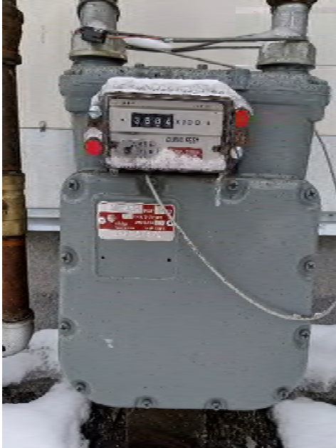
UNIT GAS METER
