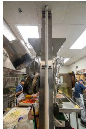
CONDENSATE DRAIN TERMINATION
