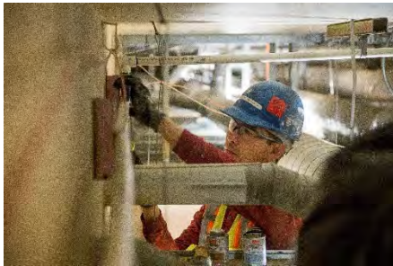
CONDENSATE DRAIN PIPING
