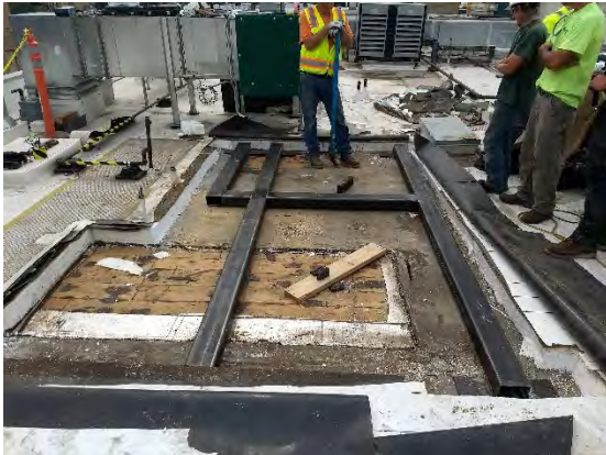
ADDITIONAL STRUCTURAL ENGINEERING, SUPPORT AND ROOFING SIGNIFICANTLY ADDED TO INSTALLATION COSTS
