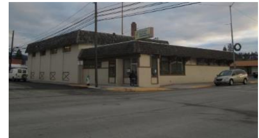
Utility Field Office – Libby, MT
