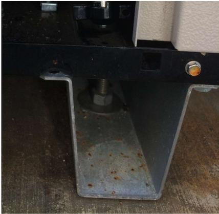
FIGURE 18 - HEAT EXCHANGER SEISMIC BOLTS
