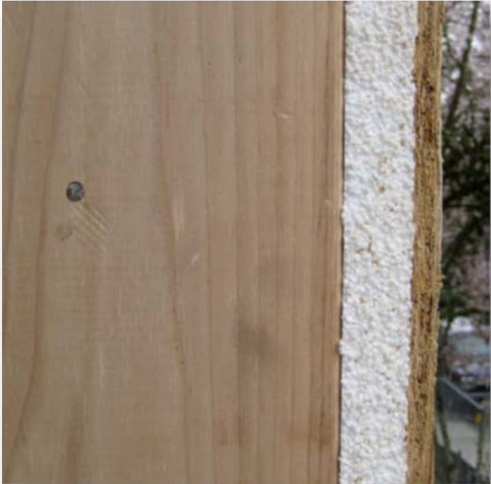
Figures 1 Cross-Section of Wall Assembly
