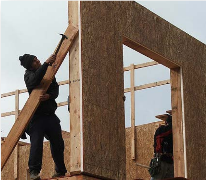
Figure 2. Construction of Wall Assembly
