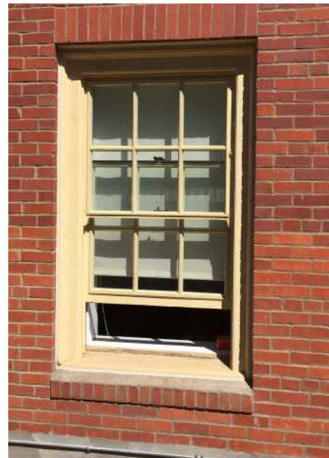
Window with SLIP attachment added
