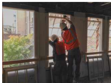
An example of a window re-installation
