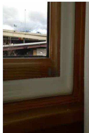
A window close-up after attachment installation. The attachment frame is in white and fits directly into the existing brown wooden frame.
