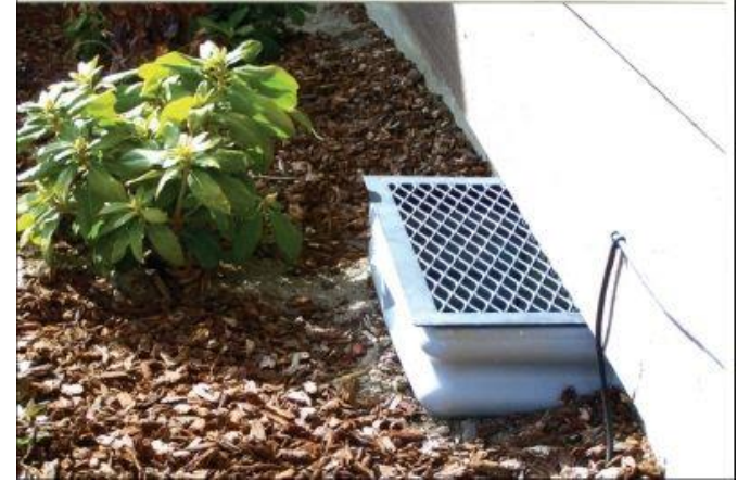
Might need a dry well
