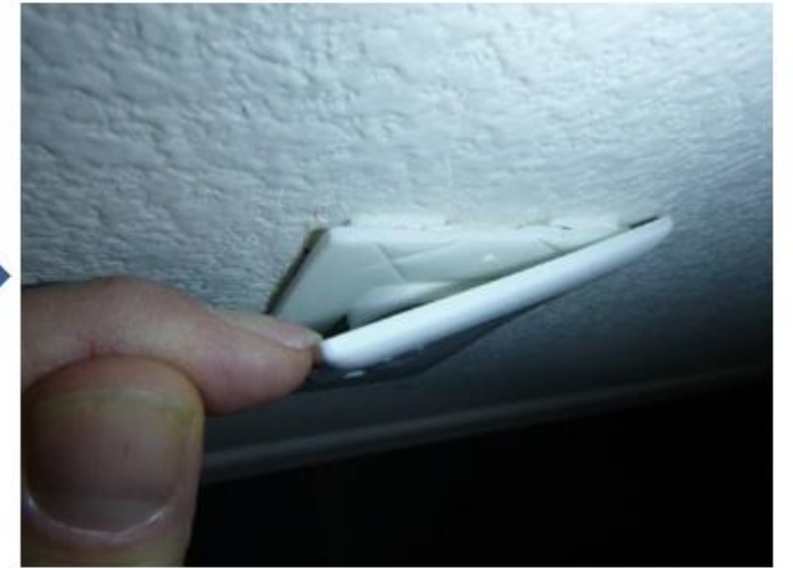
Outlet boxes get foamed in factory and include foam gasket
