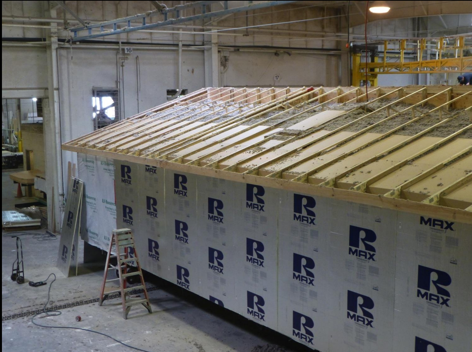
Exterior Rigid Insulation
