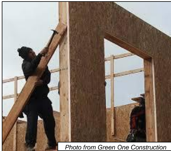
Figure 5. Framers Assembling TBS Wall
