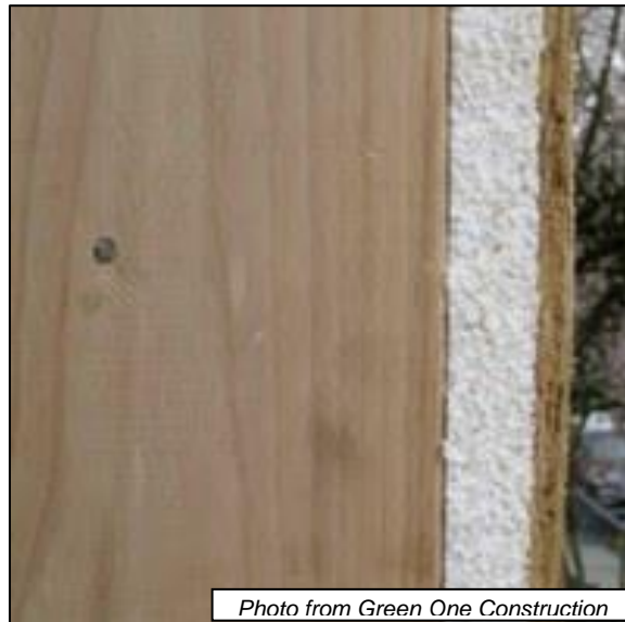
Figure 1. Thermal Break Shear Wall
