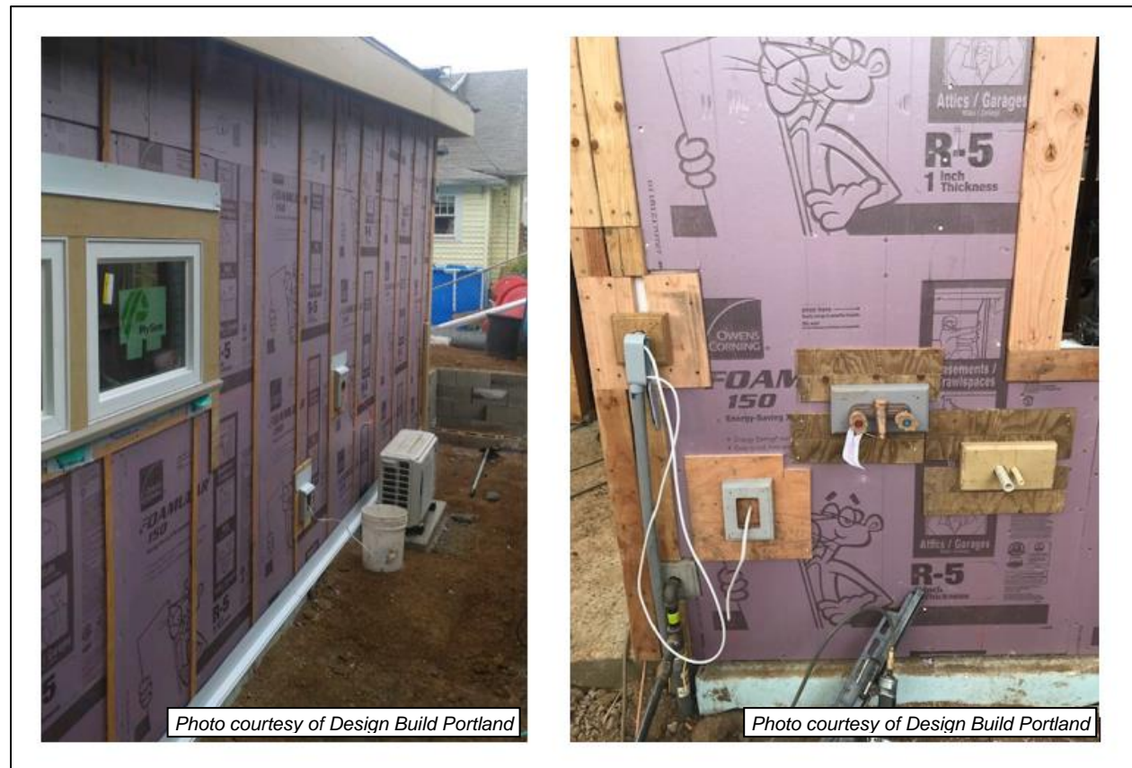
Figure 13 (left). XPS Insulation with Rainscreen Figure 14 (right). Blocking for Electrical Outlets
