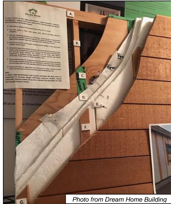
Figure 9. Design Wall Mock-Up Demonstrating Option 2 for 2x6 Intermediate Frame with Exterior Rigid Insulation
