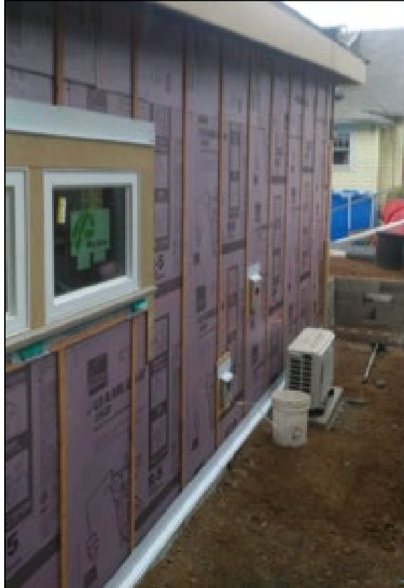
Figure 20. A completed rainscreen over exterior rigid insulation Courtesy of Design Build PDX of a
