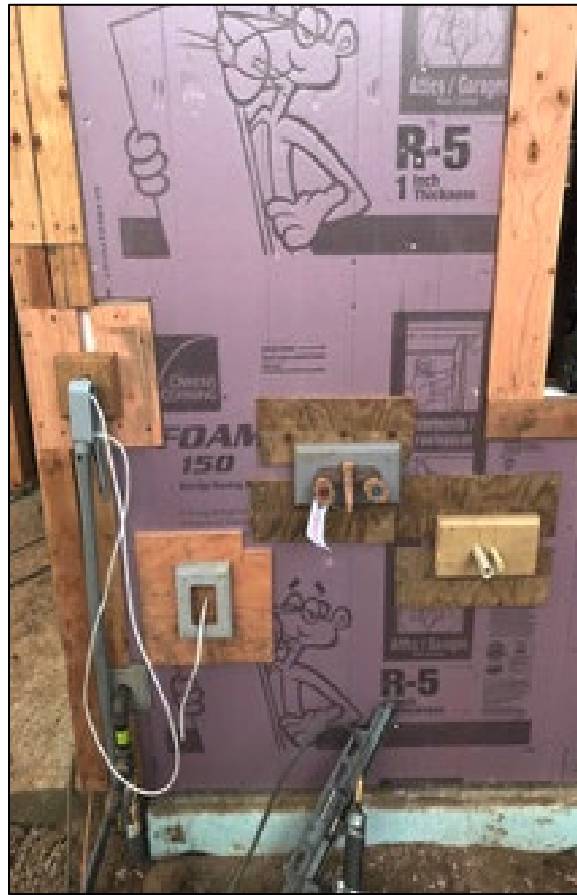
Figure 19. Wood Strapping Installation around Exterior Outlets (Image courtesy of Design Build PDX)
