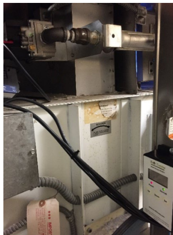
Figure 2: Bio-Therm Modulating valve and controller installed at Site in MN
