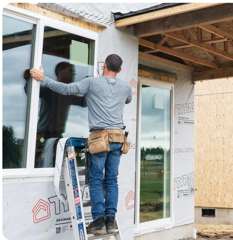
Pictured: Triple-pane window installation
