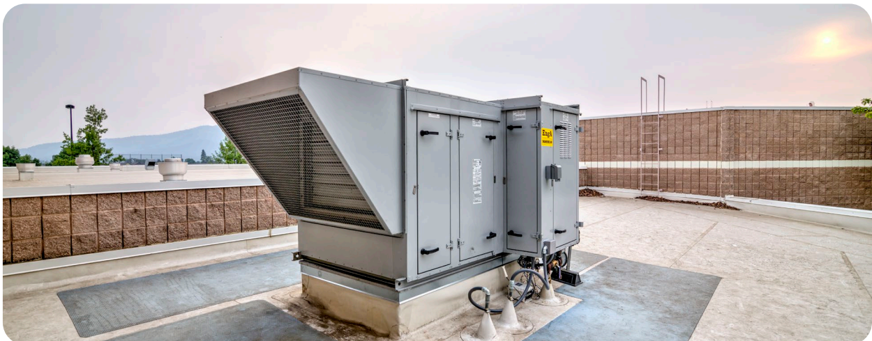
Pictured: Gas condensing rooftop unit, Post Falls, Idaho
