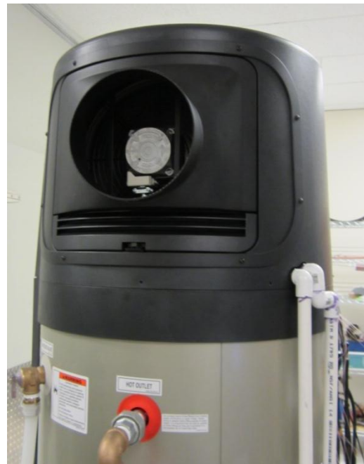
Figure 2. Exhaust Ducting Kit Attached
