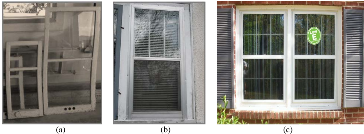
Figure 1. Evolution of Storm Window Design and Construction: (a) Traditional seasonal storm panels. (b) Aluminum-framed, self-storing storm window and screen. (c) High-performance, low-e storm windows.
