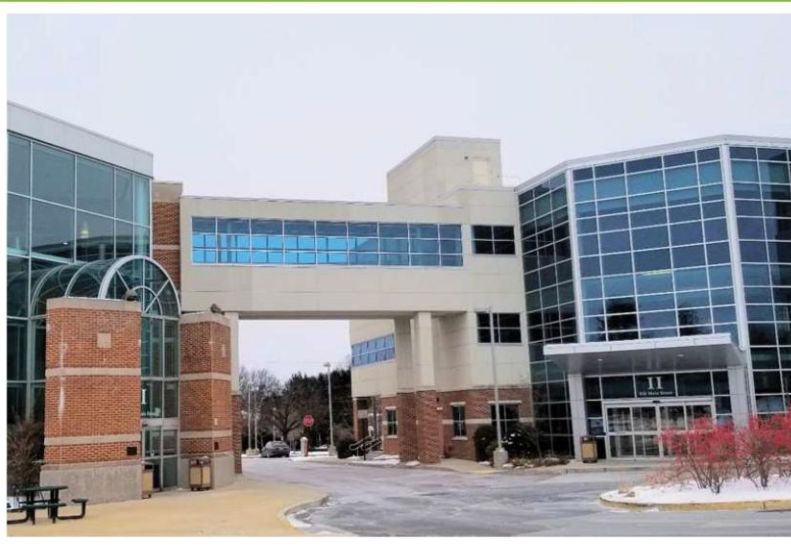
Exhibit 2-13. Buildings Connected by Walkways
