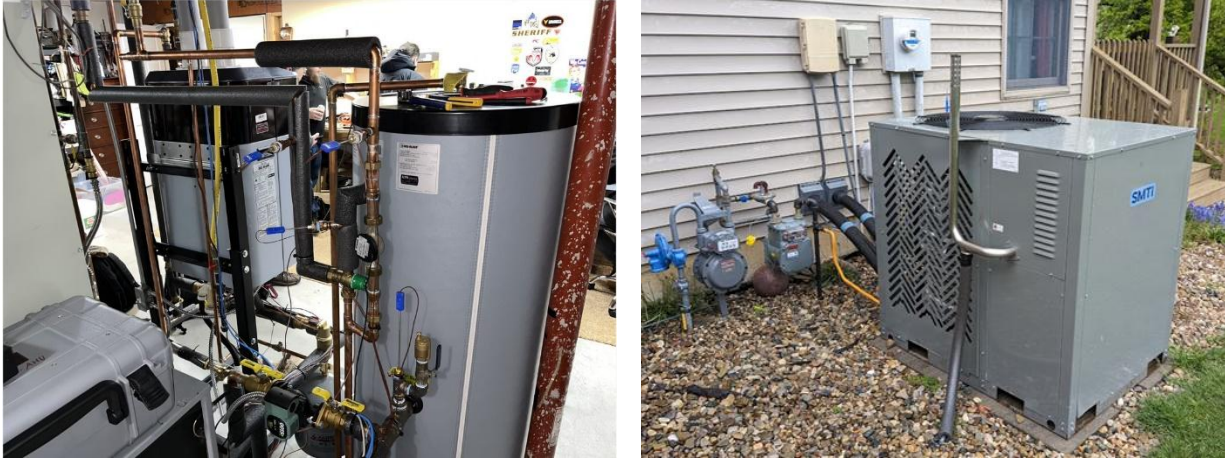
Figure 26: Single family GAHP Combi at New Carlisle Forced Air Heating Site
