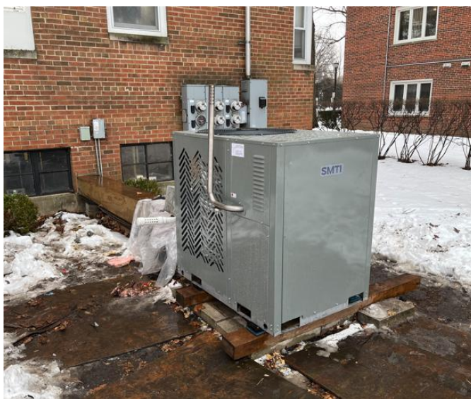
Figure 23: Evanston Multifamily Home Installation of Check Valve 2022
