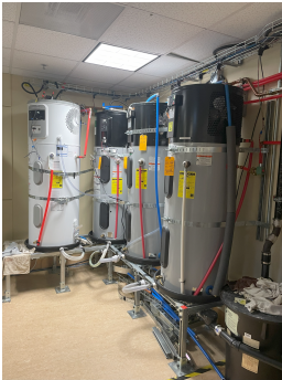
PSU PEG WH Testing Bays
