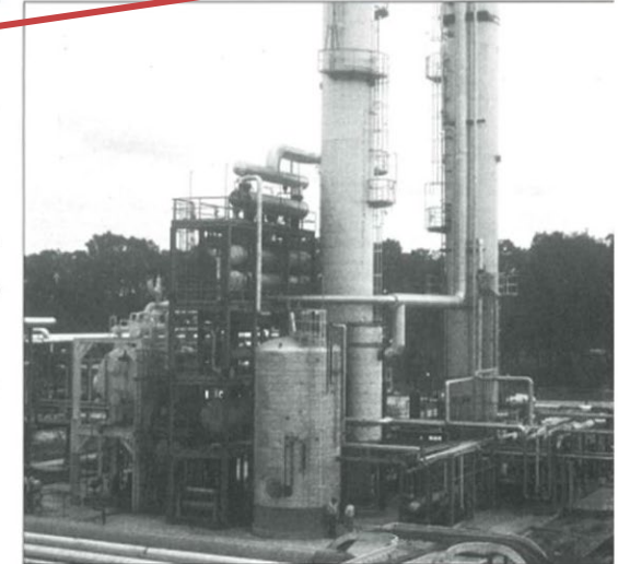
Pinch analysis identifies potential energy savings for many processes. For low-temperature, high-pressure processes, such as this nitrous oxide plant, pinch typically reduces the compressor horsepower by 20%.
